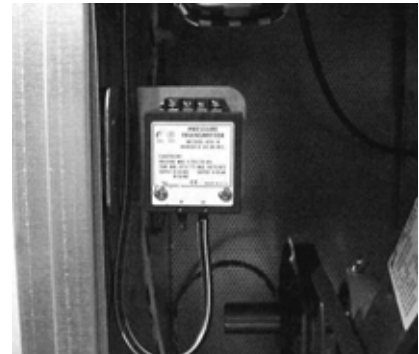
Figure 65. Piezo ring airflow measurement
